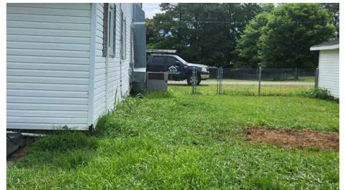
Side of house. Hard to tell with high grass. Slopes toward house
